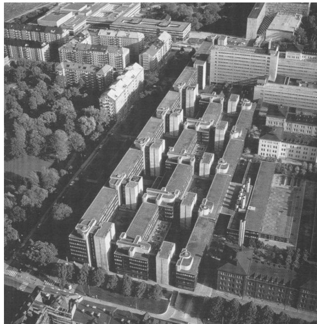
Figure 2. Aerial photo of the block Garnisonen showing the system of staircase towers as “servant spaces”. Photo Coordinator architects.
