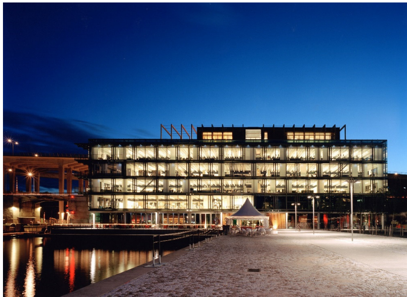
Figure 8. Katsan office block for White architects. An open office structure with glass façades facing east and west and water from the canal used for cooling. Photo White architects.
