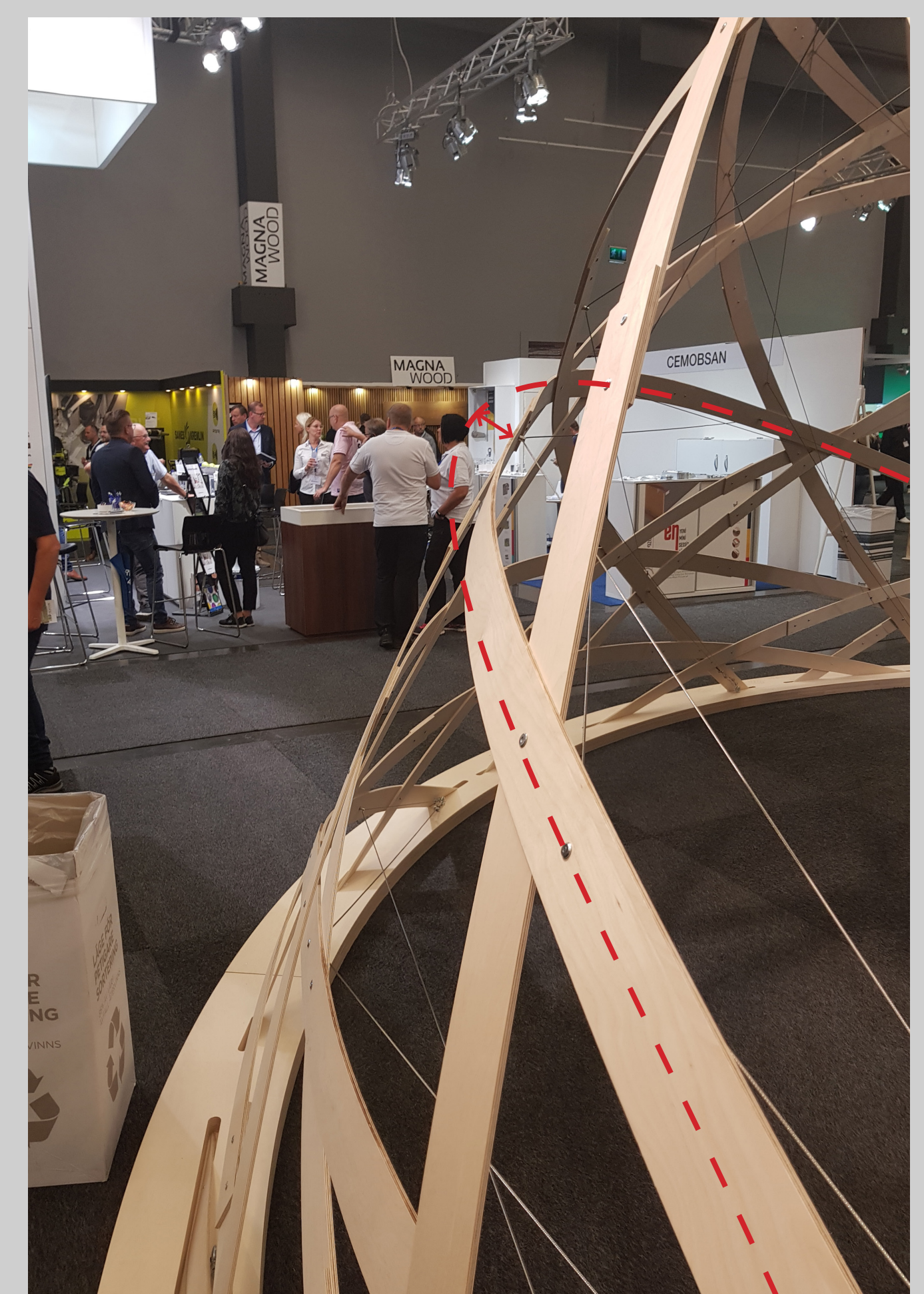
Figure 5: Lath curvature effected by pre-stress.
