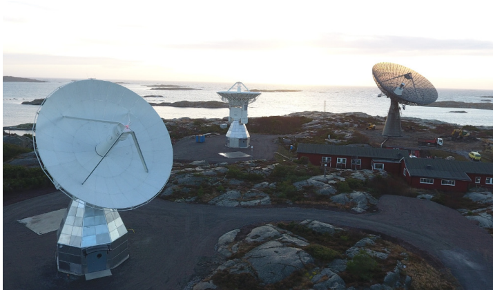
Fig. 1.1: Onsala's two 13.2 m twin telescope reflectors on the left and the 25 m telescope on the right. Image credit: Roger Hammargren, OSO.
