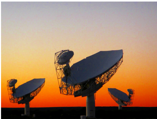
Fig. 1.2: Three of the 64 offset Gregorian reflectors of MeerKAT, each with a 13.5 m diameter, located in the Karoo desert, South Africa. Image credit: Leif Heldner, OSO.
