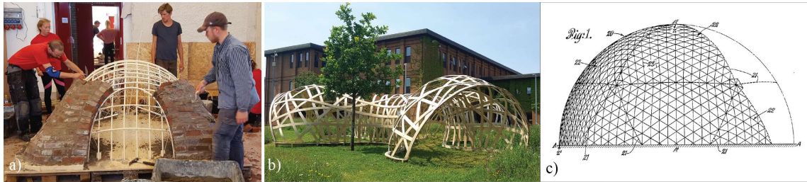
Figure 2, a) A vaulting workshop using falsework from straight plastic tubes (Adiels, [2]), b) UWE Research pavilion (Harding et al [9]) c) The geodesic dome by Buckminster Fuller (Fuller, [3]).
