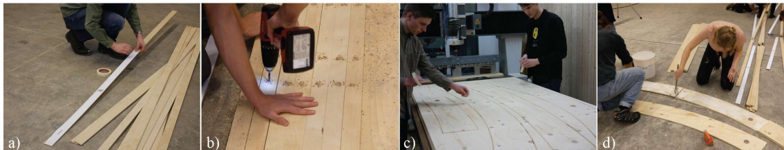
Figure 7a) taping paper drawings onto wooden strips b) predrilling marked wooden strips c) the base plates were cut out using a CNC machine d) the base plates were made of two layers 12 mm plywood laminated using glue.
