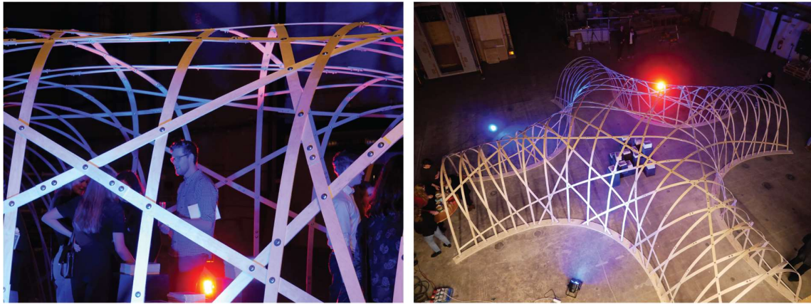
Figure 1, the result of the workshop was a geodesic gridshell built from predrilled planar straight laths.
