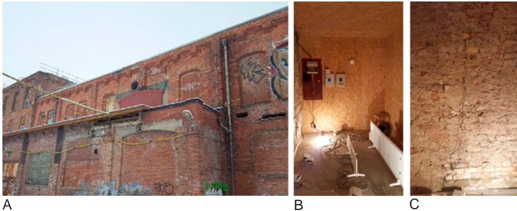
Figure 3. A) Industrial building from 1896 south of Gothenburg to be insulated on the interior with VIP, B) The test room inside the industrial building, C) Sensors in the external brick wall. Photos: Pär Johansson.
