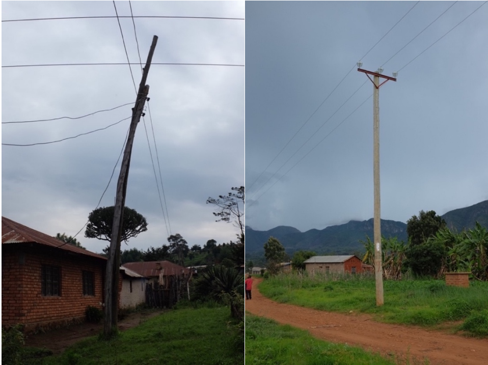
Figure 4 Examples of cases with poor-quality equipment (left) and good-quality equipment (right).
