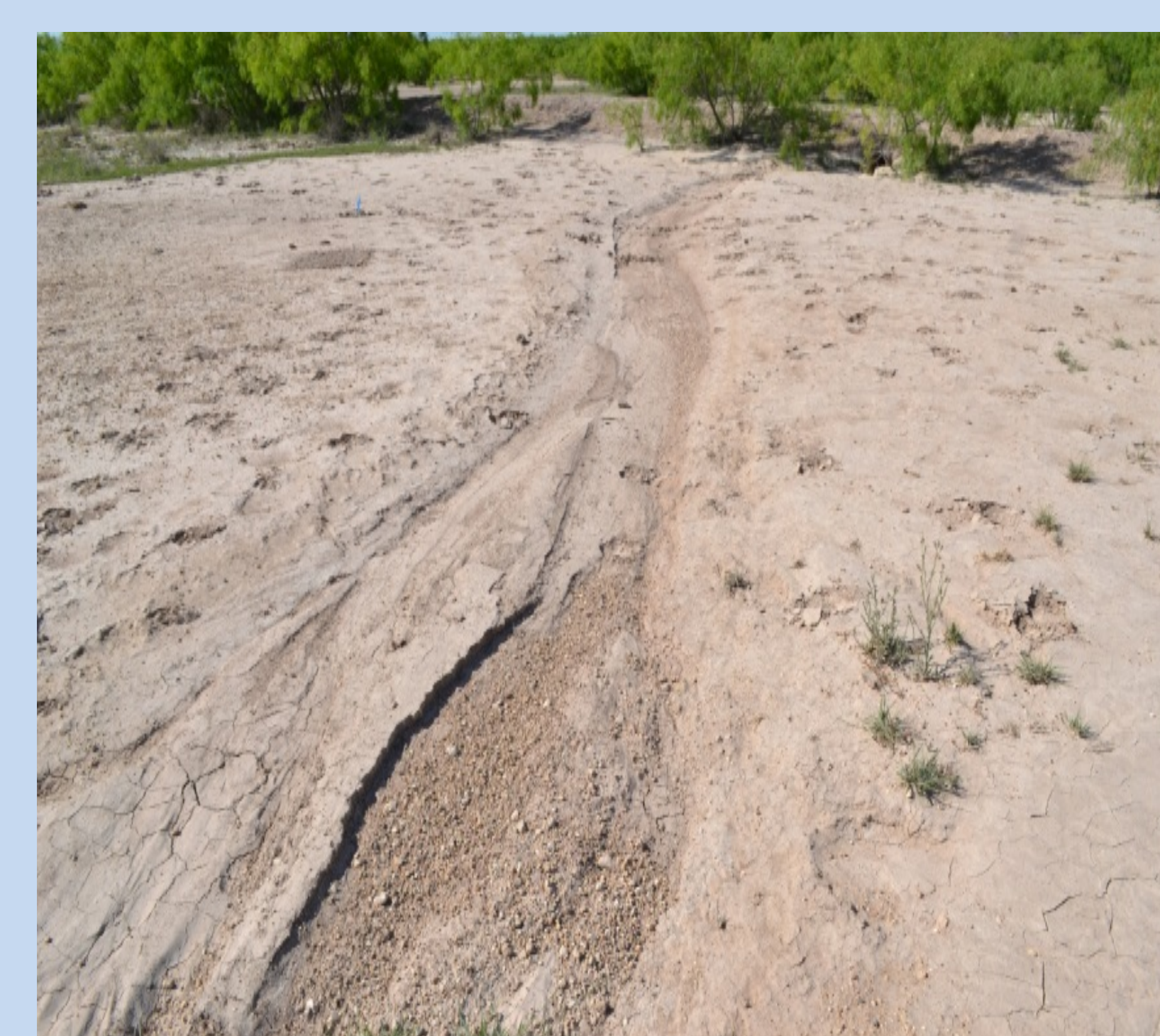
Figure 5: Photo Showing Salt Crust, Mudcracks, and Erosion
