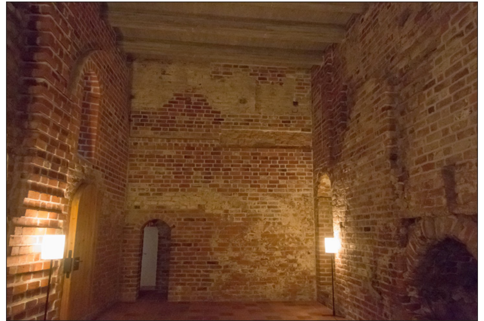
Image 1. The current form of the Knights' Hall. Remains of the vaults are visible in the walls.
