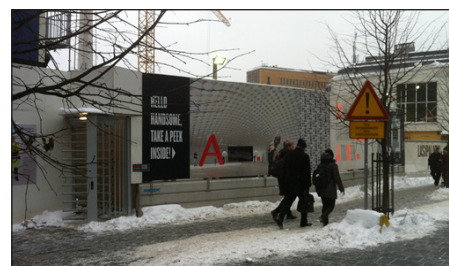
Image 3: Installation integrated with the construction site fence as a viewing hole
