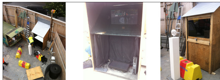
Image 2: Building of the installation at the final location in construction site
