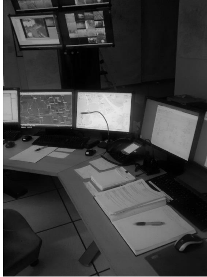
Figure 1. Technicians' workspace (authors' own).
