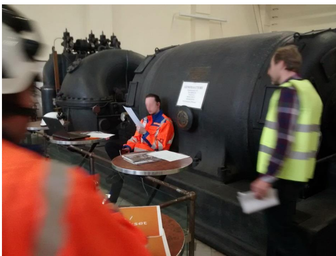
Figure 4. Technicians around an old generator from ca. the 1930s
