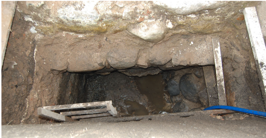
Fig. 3. Town wall in the excavation pit in Vabaduse Avenue (according to Bernotas 2010a). Photo by Rivo Bernotas.
