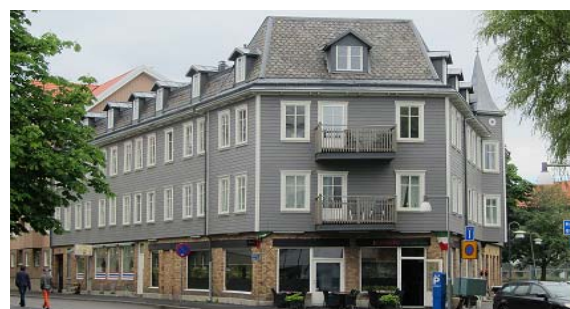
Fig 2: The building at Brämaregatan in its current state, after 2010.
