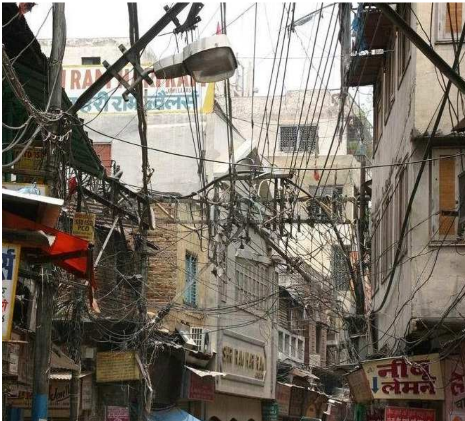
Figure 7. Overhead lines in use at urban area in India.
