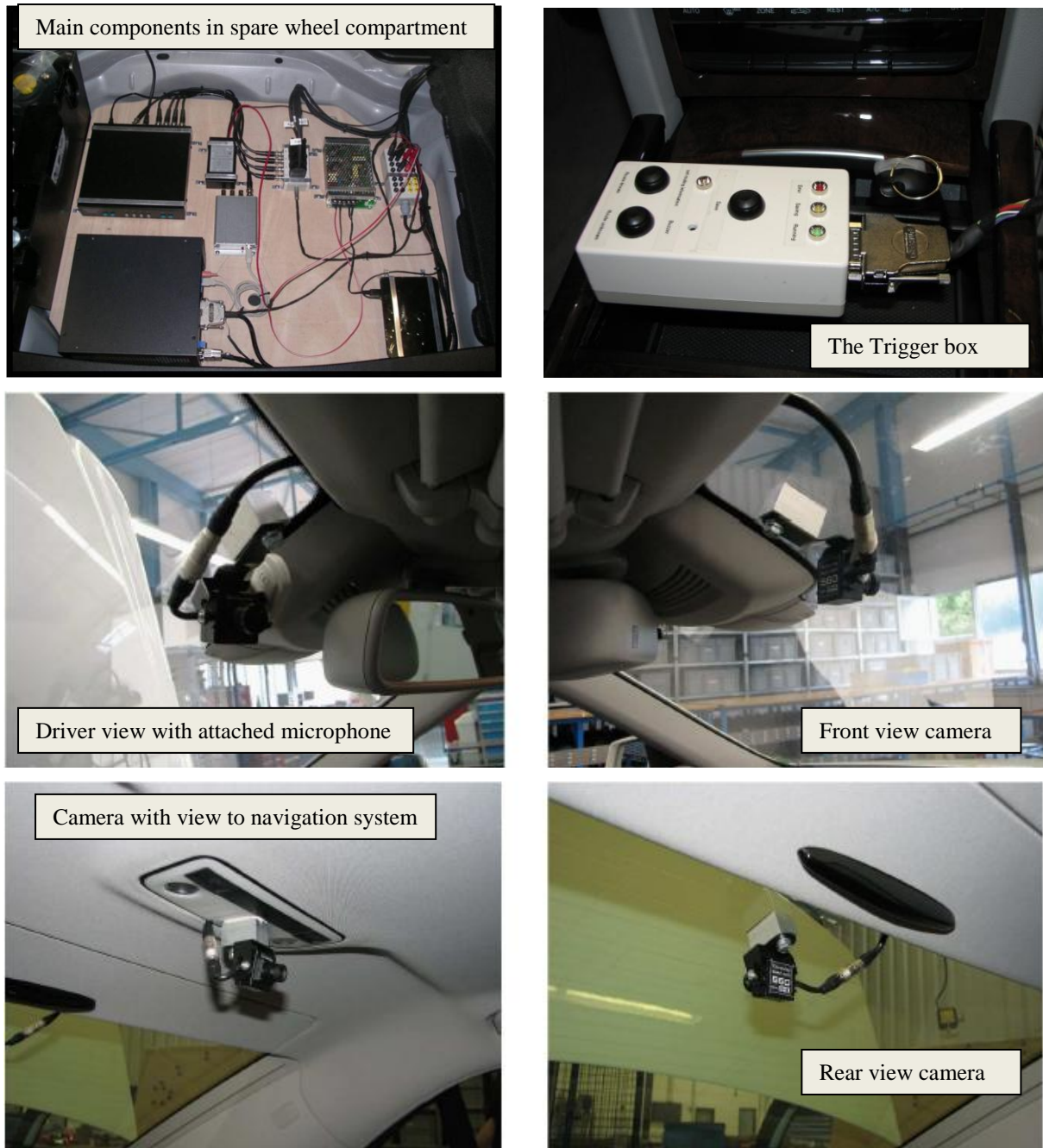
Figure 23: Placement of DAS in a Daimler vehicle. This figure is adapted from euroFOT-Daimler installation guide.
