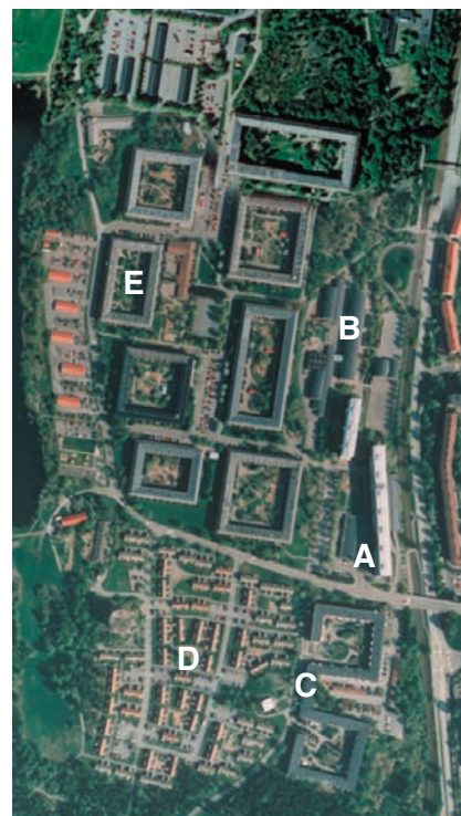
Fig. 8. Air-photograph of Northern Biskopsgården.
