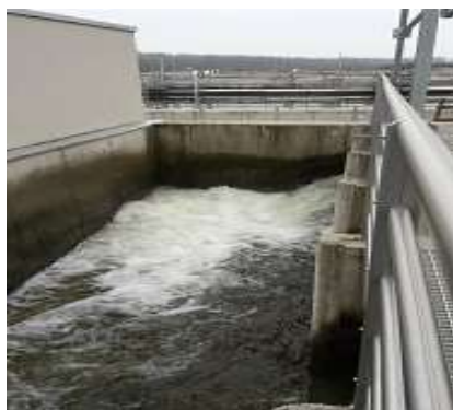
Slika 7. Crpljenje efluenta u recipijent Fig. 7. Point of the effluent embarking into the recipient
