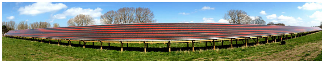
Figure 5.1.: Panorama photograph of the first row of the solar park with six parallel installed solar cell modules of 100 m length each. Adapted from [99] © 2013 WILEY-VCH Verlag GmbH & Co. KGaA, Weinheim.
