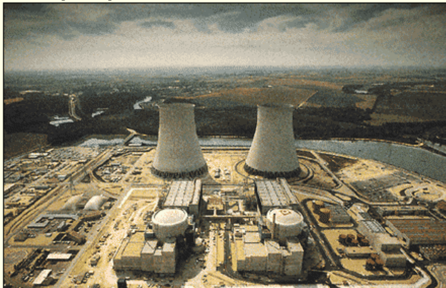
Nuclear power plant
