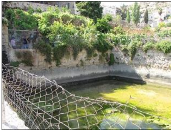
Fig. 7.7: A modern plastered pool at Battir, built on the foundations of older one as part of a traditional irrigation system.
