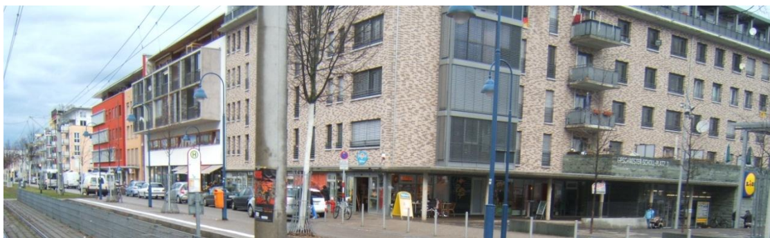
Fig. 6.22 Retail at Geschwister-Scholl Platz, Rieselfeld
