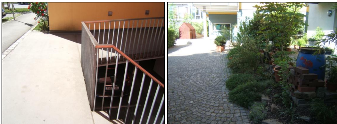
Fig.8.10 Open access parking (a) and soft boundaries around residential property (b)
