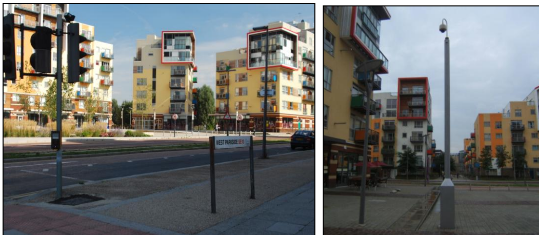
Fig.8.12 Millennium Village Central Square (A) Showing Busway, and (B) CCTV Camera
