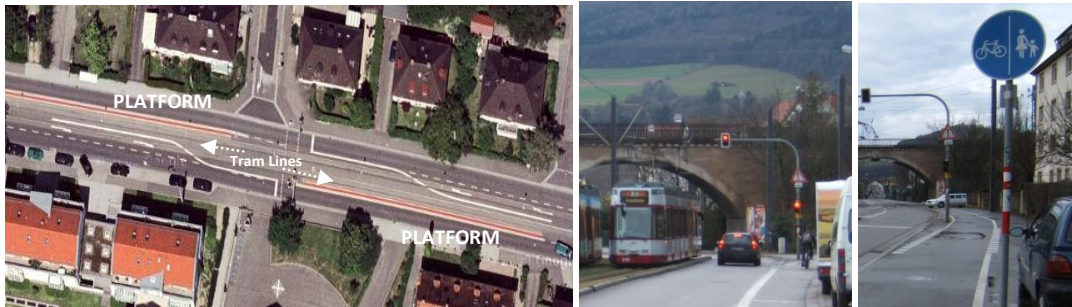
Fig. 6.10 Car-Alternative Priority (a) Carriageway Platforms (b) Priority Signalling (c) Signal By-Pass for Cyclists
