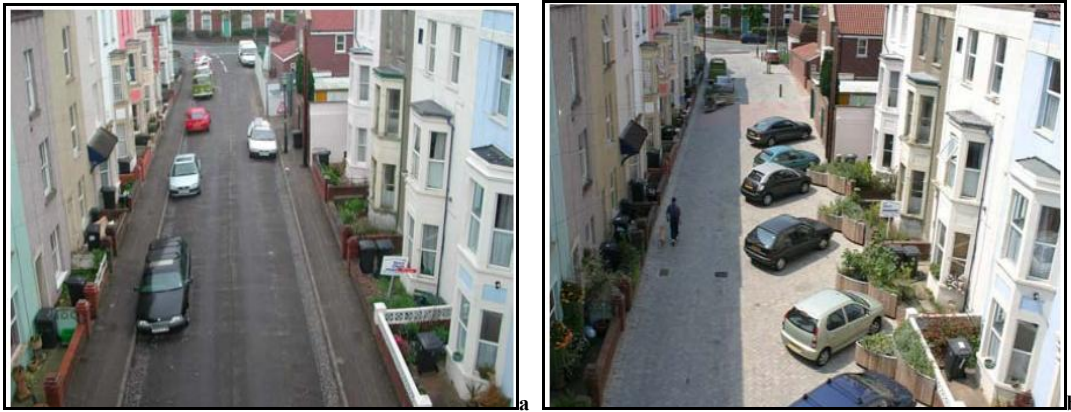
Fig. 3.9 Millford Street, Bristol: before (a) and after (b) home zone re-modelling (Chatterjee, 2009)
