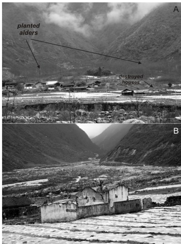
Fig. 1. The debris flow fan under study, (A) – the village is located on the debris flow fan and the planted alders are marked with arrows, (B) – one of the houses destroyed by debris flows.
