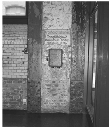
Photo 5. Functional details of the former power plant become decorative elements in the new space, September 2017 (Magdalena Abraham-Diefenbach)
