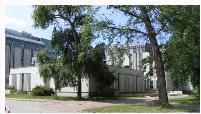
Figure 1: The Heavy Ion Laboratory building, North side.
