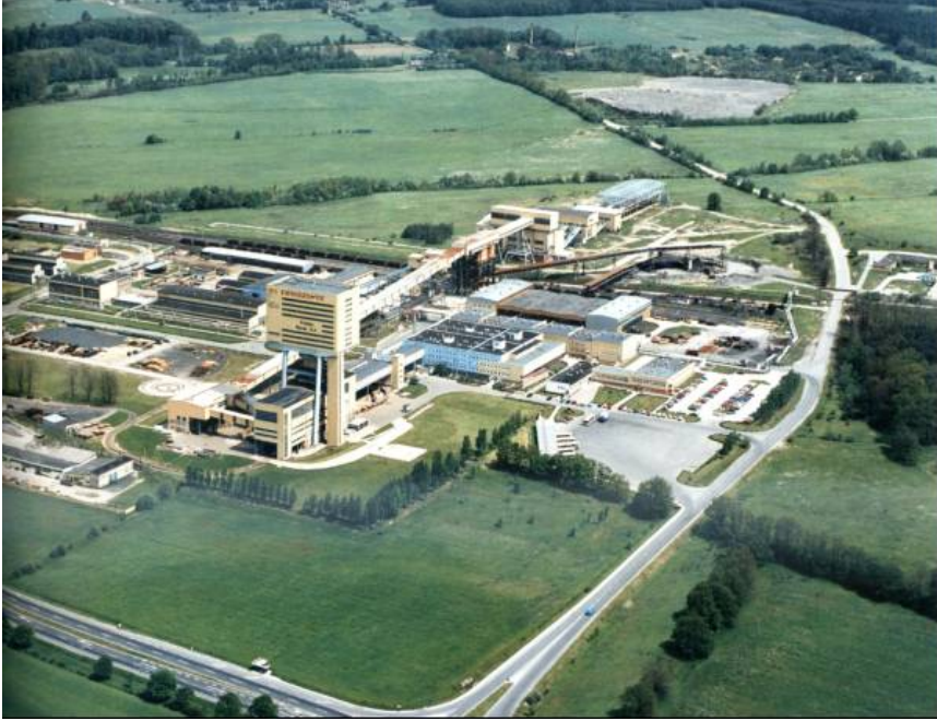
Fig. 2. Photo of the Polkowice–Sieroszowice surface buildings.
