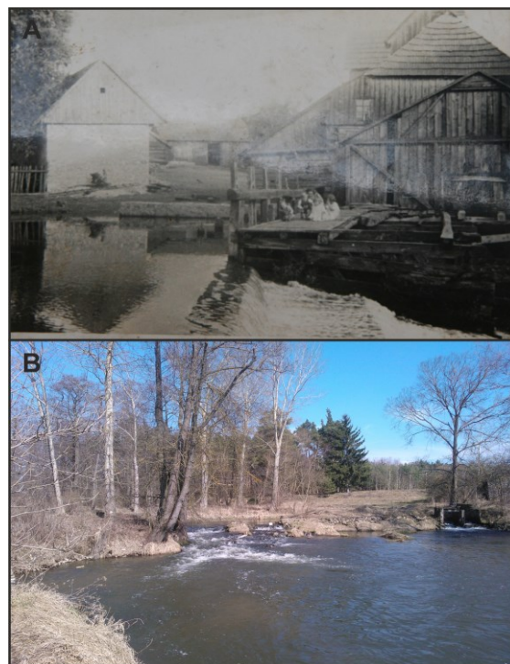
Fig.5. A – A photo from the 1950’s showing the dam and the mill building. B- The interrupted dam, with the remains of the weir on the right hand side and the eroded bank of the left hand side of the river channel
