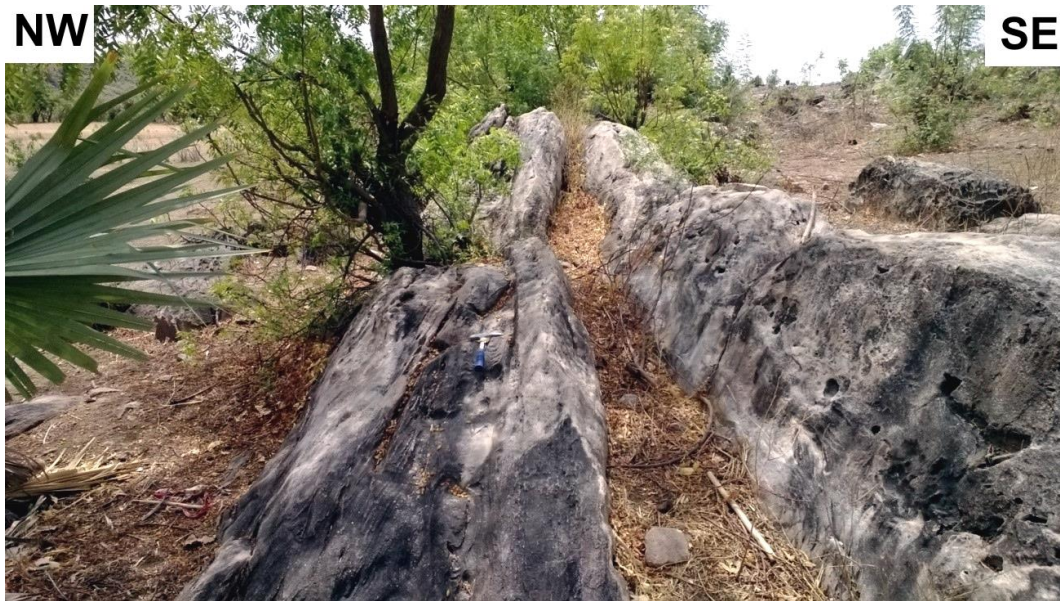
Plate 1. NE – SW trending fault being a part of the Kaltungo Fault Zone within the Upper Bima Formation at Lallapido (location of the site: N09° 43' 13" and E01° 08' 58").
