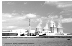
Coal Power Plant
