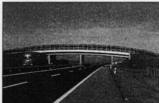
Photo 3. 151.709-km Game Bridge of the M1 Motorway
