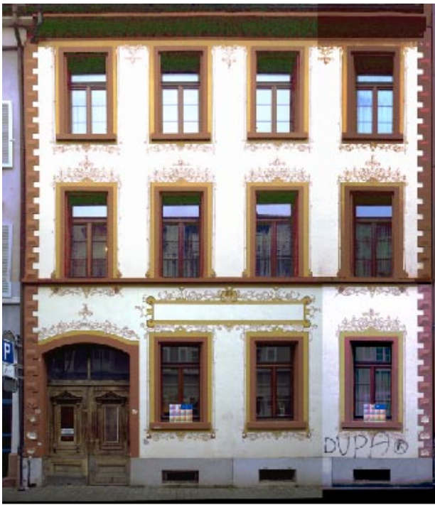
Figure 8: Mosaicing of a plane facade consisting of four images rectified and joined together.
