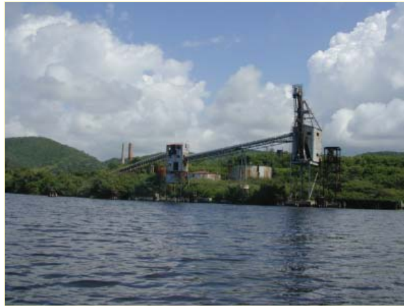
Abandoned industrial facility on the shores of Guanica Bay.
