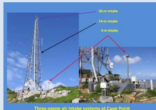
Three ozone air intake systems at Cape Point
