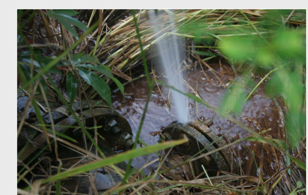
Dilapidated pipeline
