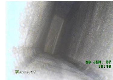
View into the cooling channel
