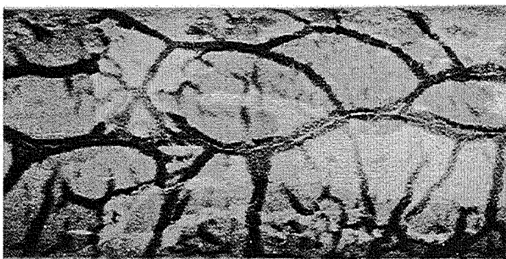
generation of through-wall cracks
