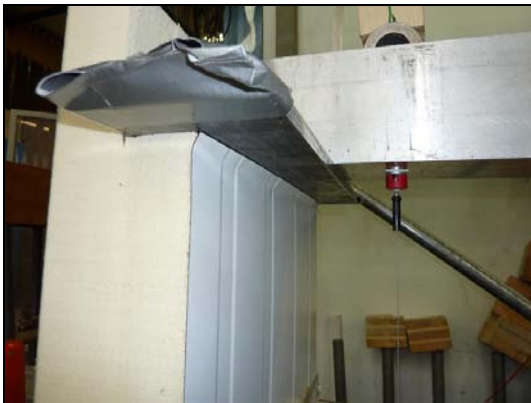
Failure of the stressed face
