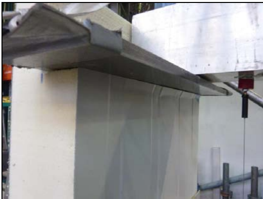
Failure of the stressed face
