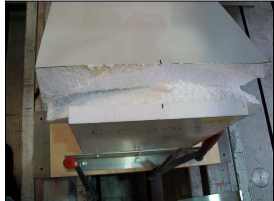
failure of core material
