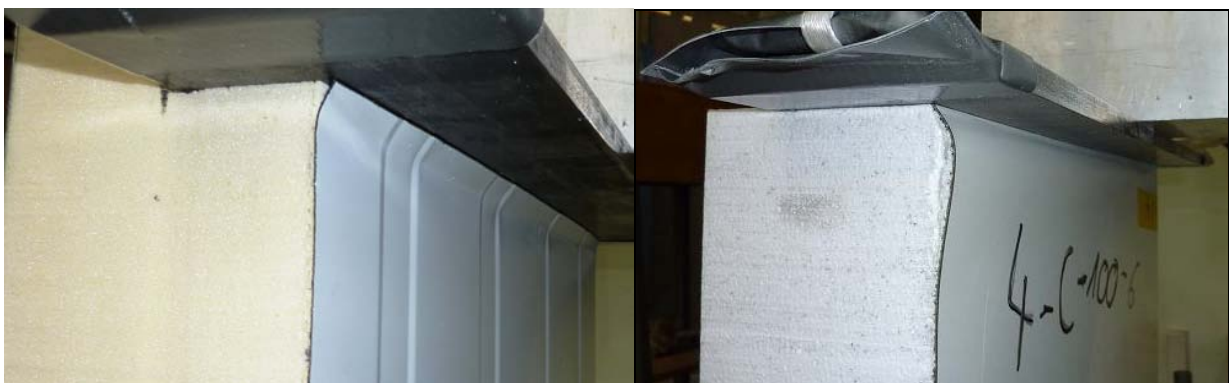
Fig. 5: Local failure at load application area
