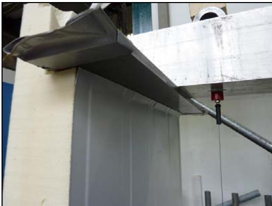
Failure of the stressed face
