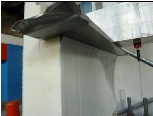
Failure of the stressed face
