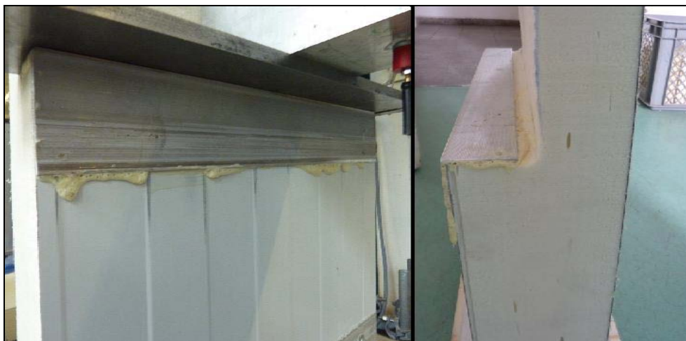
Fig. 16: Wall panel with glued angle for improvement of the load application area
