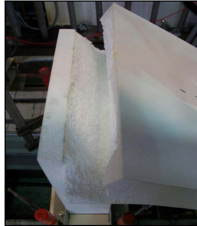
failure of core material
