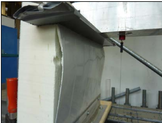
Failure of the stressed face
