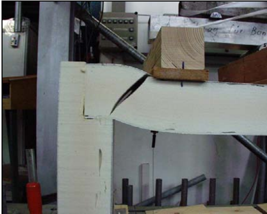
shear failure of the ceiling panel
