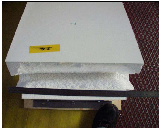
failure of core material
