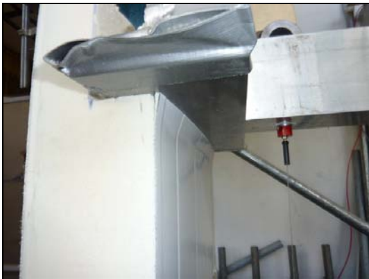
Failure of the stressed face
