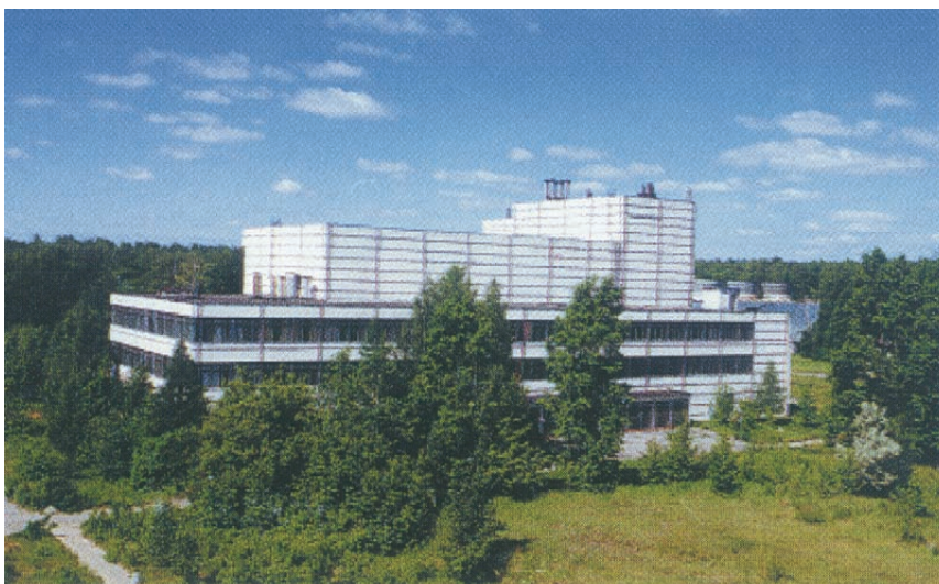
Fig. 2-4 Reactor building of BOR 60.
