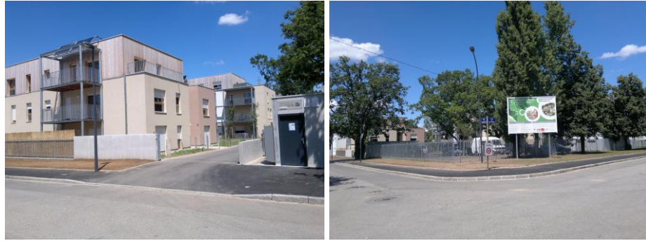
Figure 80 New constructions at rue du Progrès and rue de Quimper on the site of the former ‘420’ in July 2012
