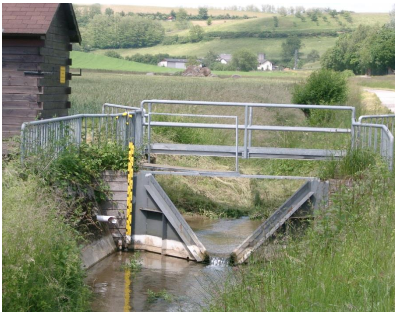
Gauge station in the Weierbach catchment
