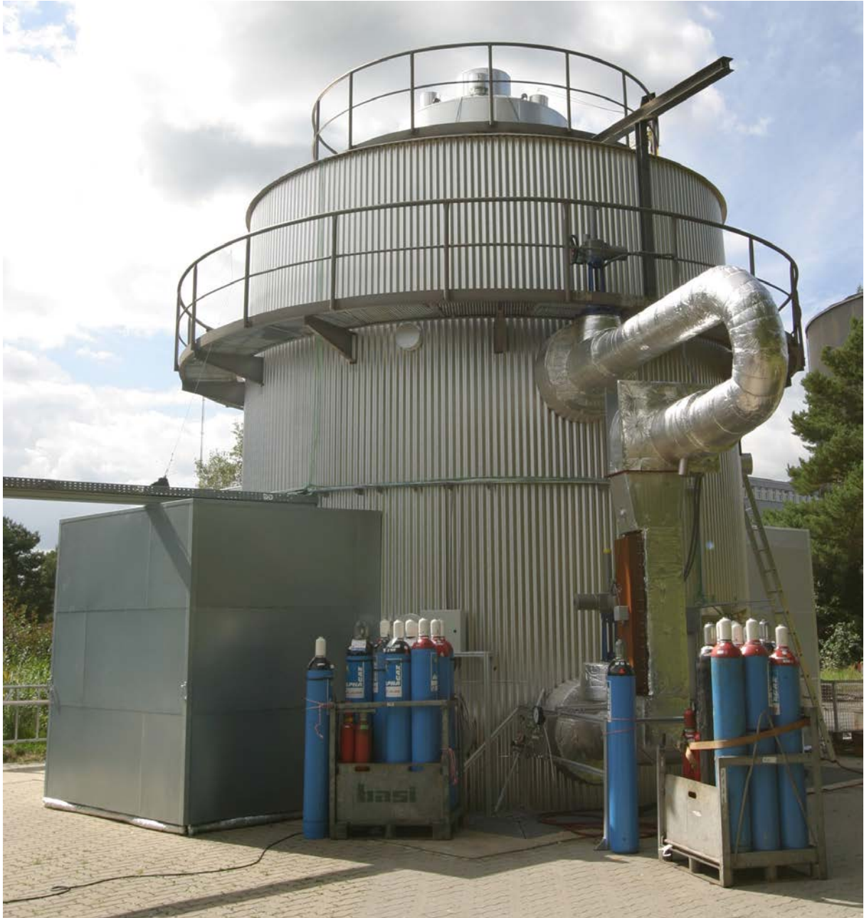
Fig. 3. Pressure vessel A2 with insulation and heating equipment
