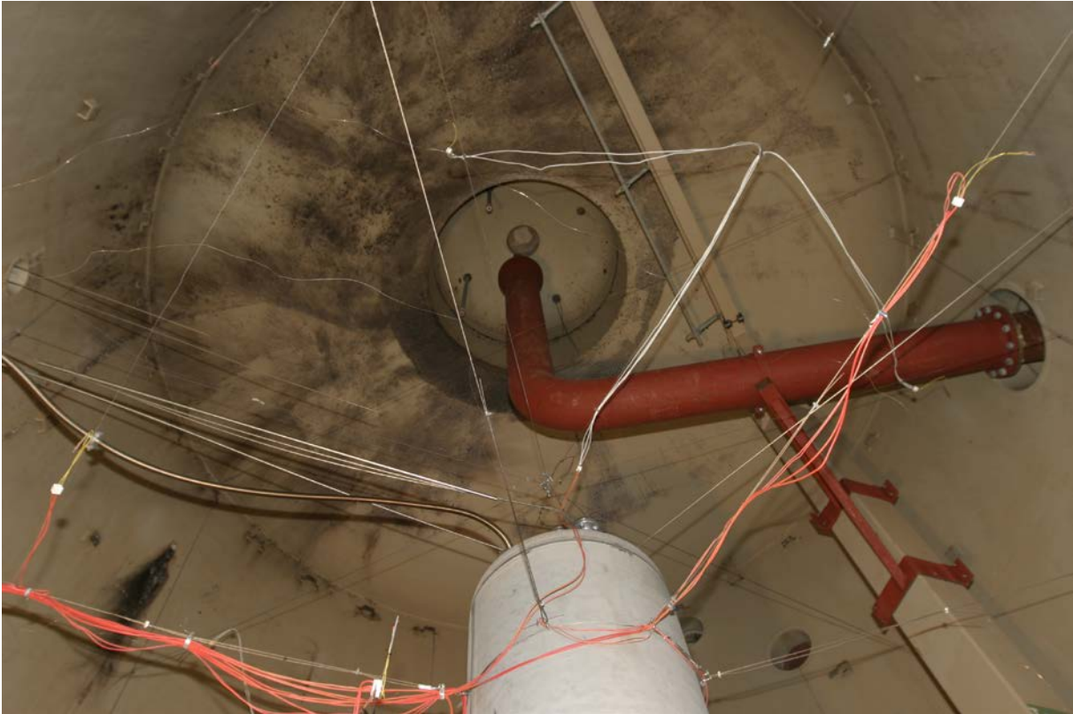
Fig. 4. Suction pipe of air heating equipment
