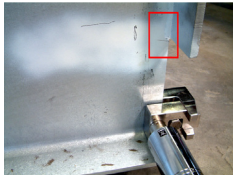
(b) Clamped transducer and marked crack location
