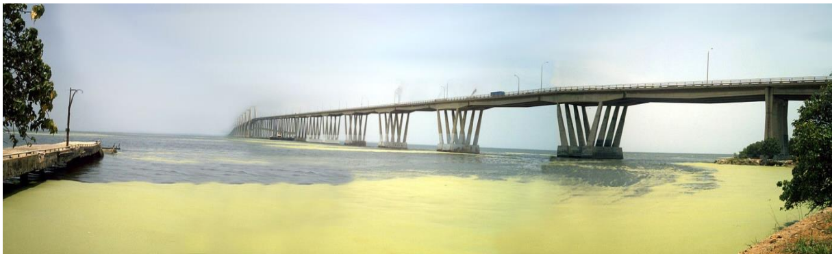
Figure 2.4 - bridge of Lake Maracaibo (Wikipedia, 2015)
