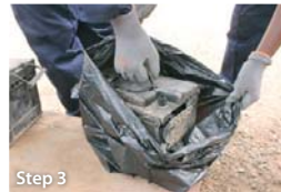
Step 3 Pack damaged batteries in heavy weight poly-ethylene plastic bags
