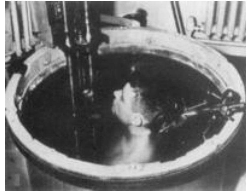
First "USCT" device (Holmes et al., 1954): Slice image of the neck, compounding device
