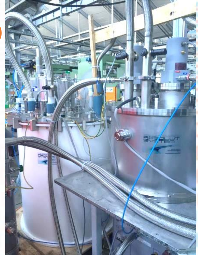
20K cold box & LN2 distribution box at customer premises
