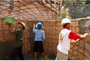
**Fig. 3** Transport of the prefabricated reinforcement cage to the cistern foundation which has been treated with a screed on a decoupling layer of old cement bags before (*top*) and application of the inner mortar layer (*bottom*)
