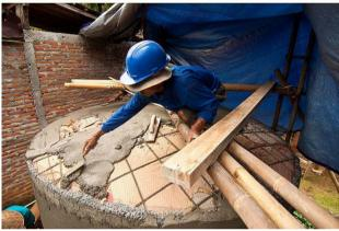
**Fig. 4** Application of the outer mortar layer (*top*) and application of the mortar on the ceiling (*bottom*)
