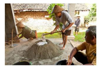
Fig. 2 Mixing of the mortar in-situ
