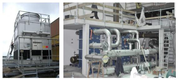
Fig. 1.6.4. 5 MW cooling tower (left) and cooling pipes in FULGOR hall (right).
