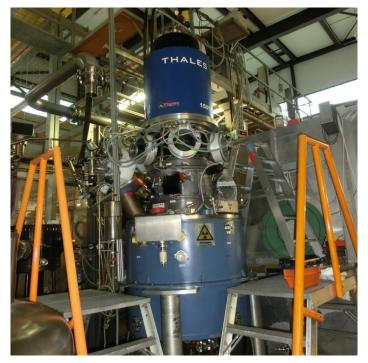
Fig. 1.2.2: First industrial ITER gyrotron after final installation at KIT in the OI Magnet.
