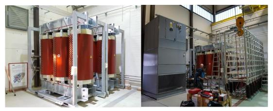
Fig. 1.6.2: Left: Two 6.5 MVA transformer installed at FULGOR hall. Right: Ventilation cabin and rack for electronic modules.
