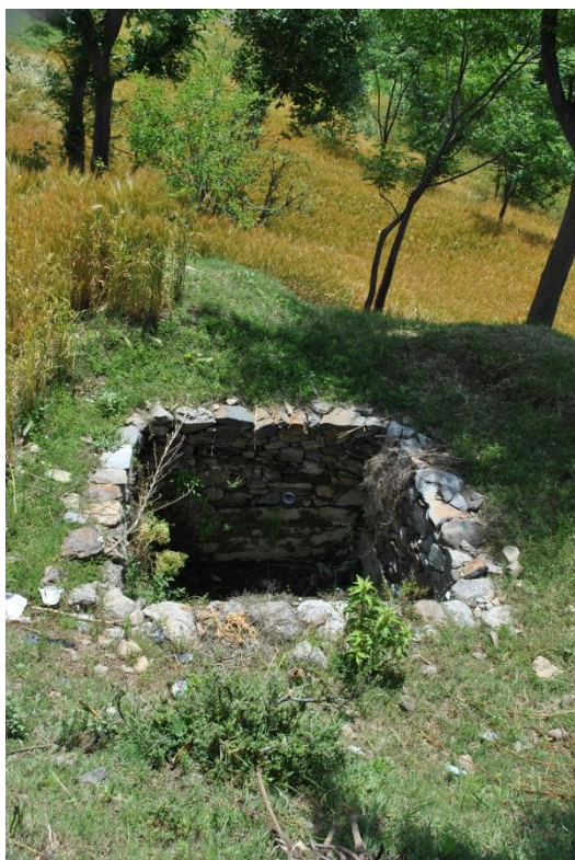
Figure 4.7 An under construction (left) and operational (right) soakage pit from village Basala.
