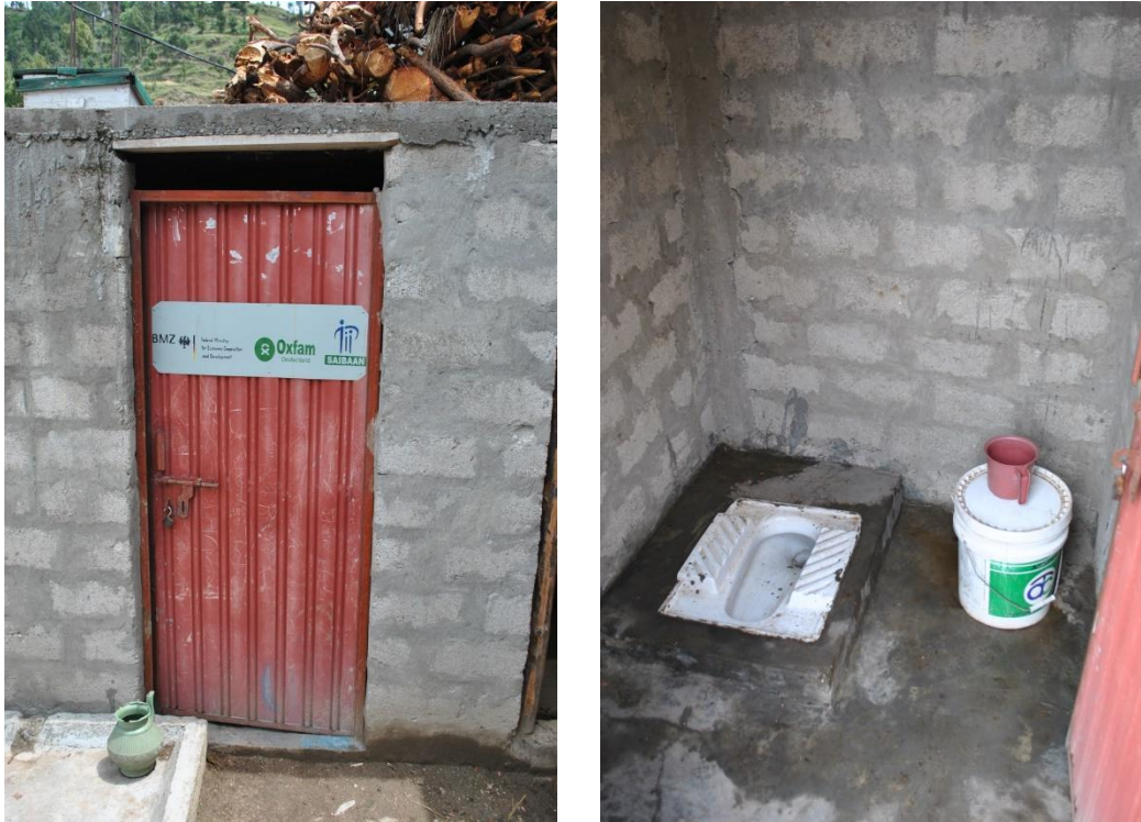
Figure 4.2 Simple pour flush latrine fitted with a squat toilet (outside and inside) in Village Basala.
