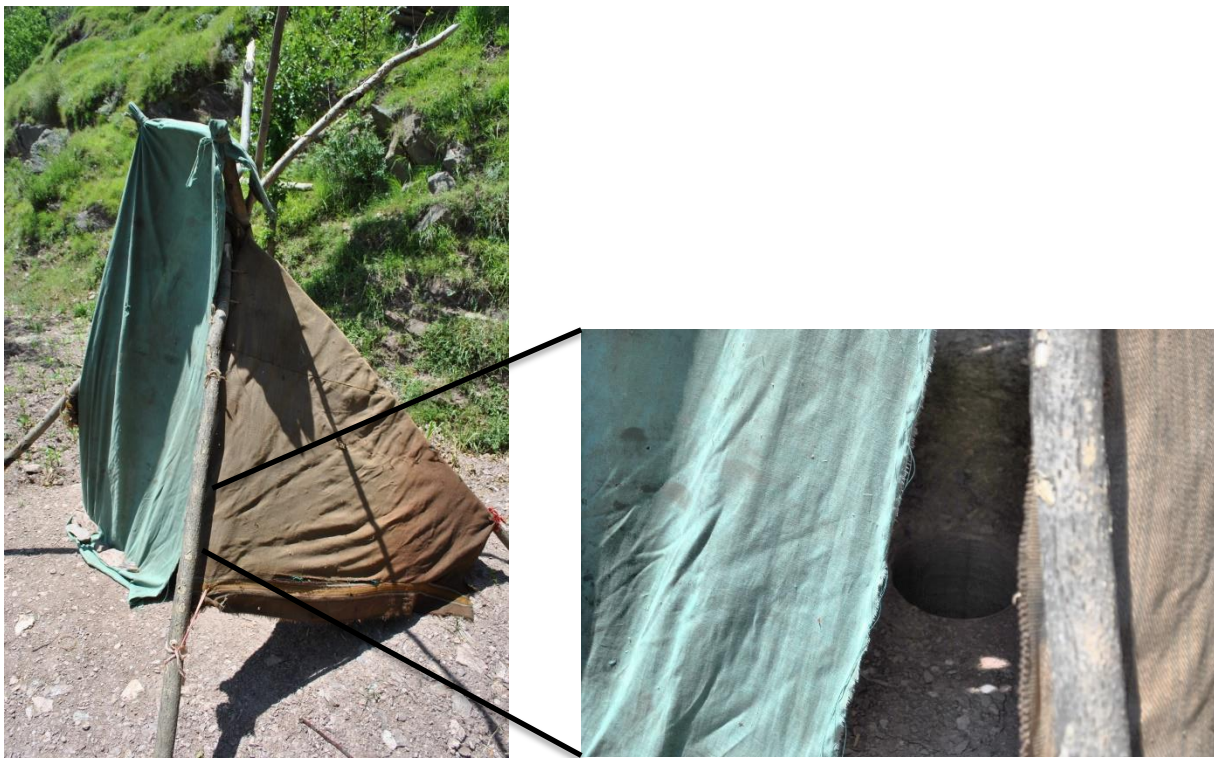
Figure 4.5 Actual pictures of a simple pit latrine from the study area (Naka Guldar). As seen in the close-up of the actual opening, no slab is present on the pit.
