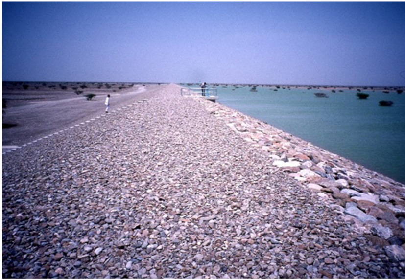
Fig. 6 Ahin recharge dam on the Batinah Plain, Oman, constructed in 1994, is a large dam (crest length 5,640 m, crest height 8 m) with a detention capacity of 6.8 Mm 3 . This is one of the 43 recharge dams, with an aggregated capacity of 95 Mm 3 constructed in Oman during the period 1985–2011 (Oman MRMWR 2012). Their purpose is to enhance aquifer recharge primarily to support irrigation; and also to protect the
