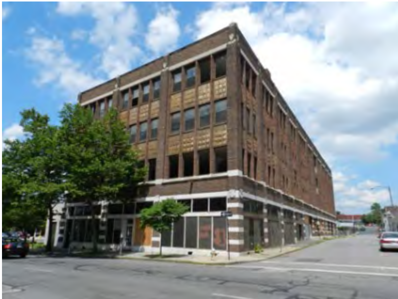
Figure 25: Willys Overland Building post gas explosion, Springfield, MA.
