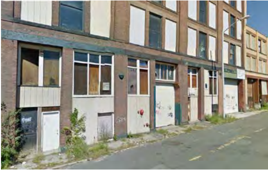
Figure 50: Current condition of Collins Building25
