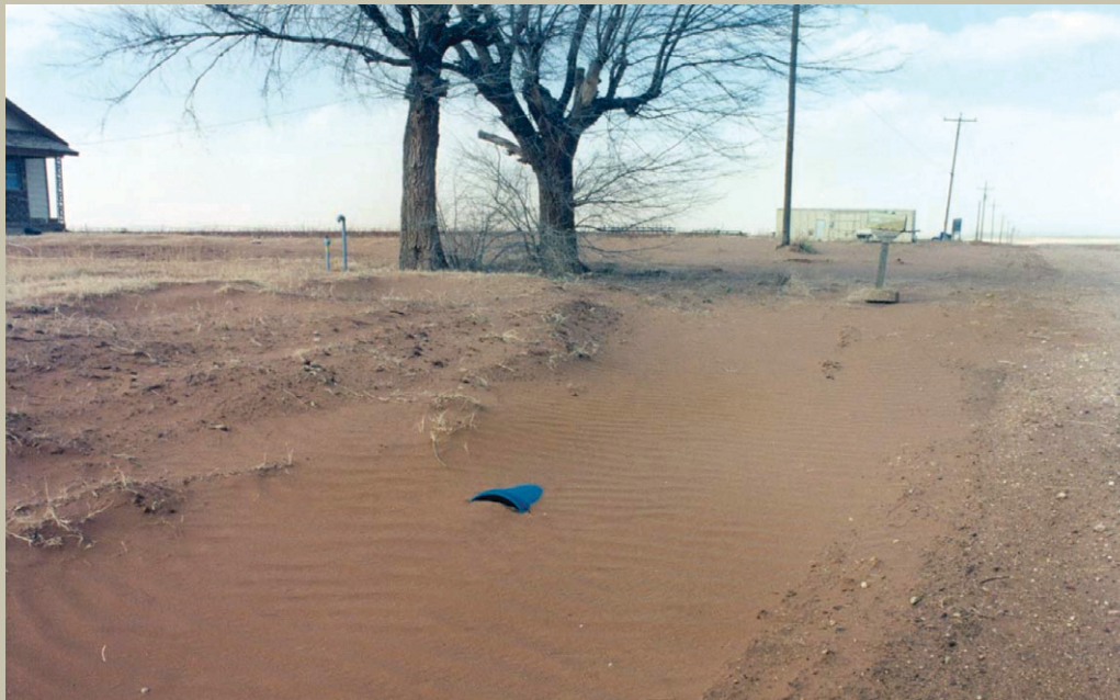
Fig. 14|4. Drainage ditch filled with sand following a severe dust storm in west Texas.
