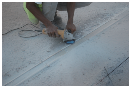
Figure 2.9. Grinding excessive grout
