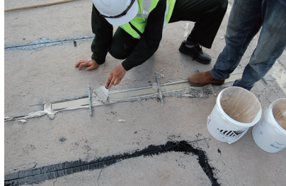
Figure 2.8. Grouting the sensor
