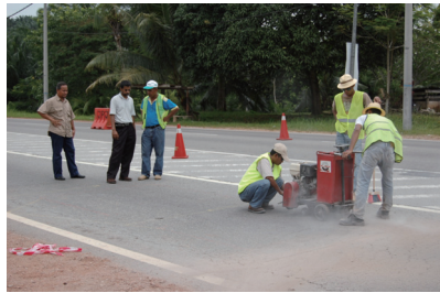
Figure 2.6. Dry cut pavement slot
